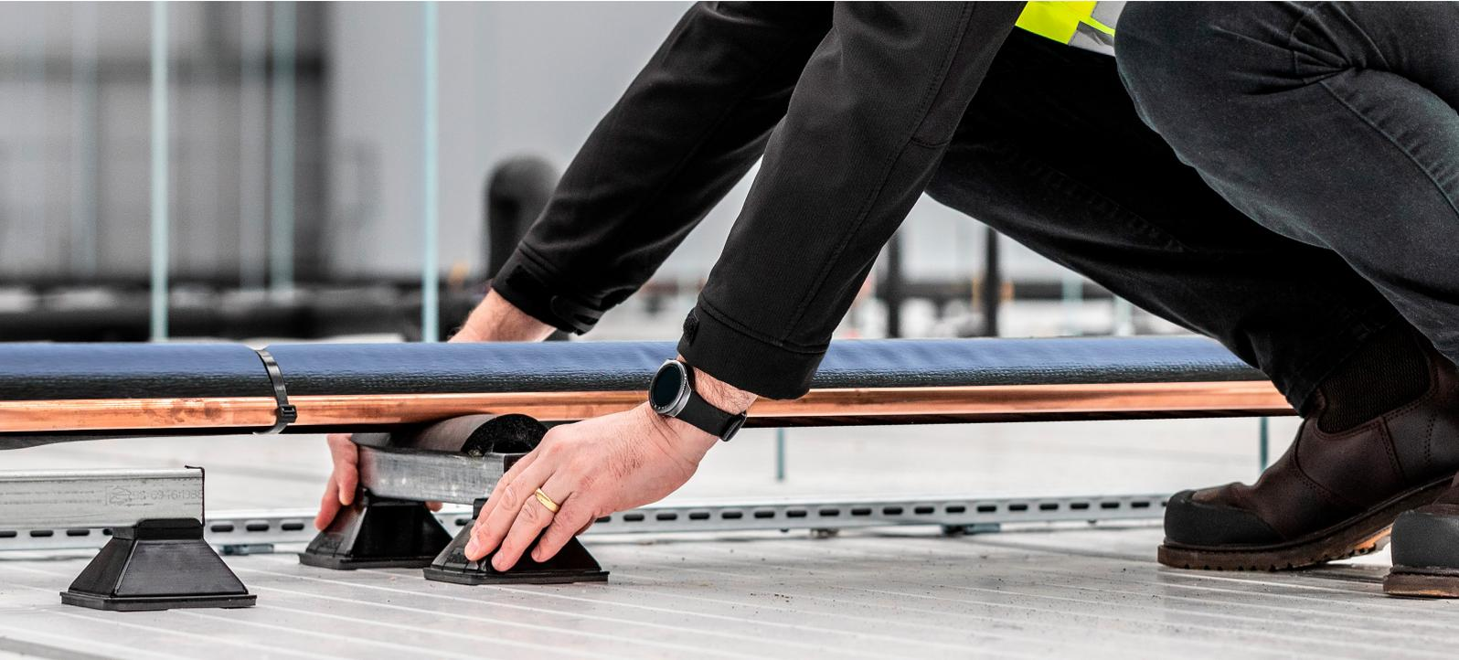
PVC Coated External Grade Insulation. External pipework needs to be insulated in a tough PVC coated weather protected covering to avoid UV degradation and animal damage.
